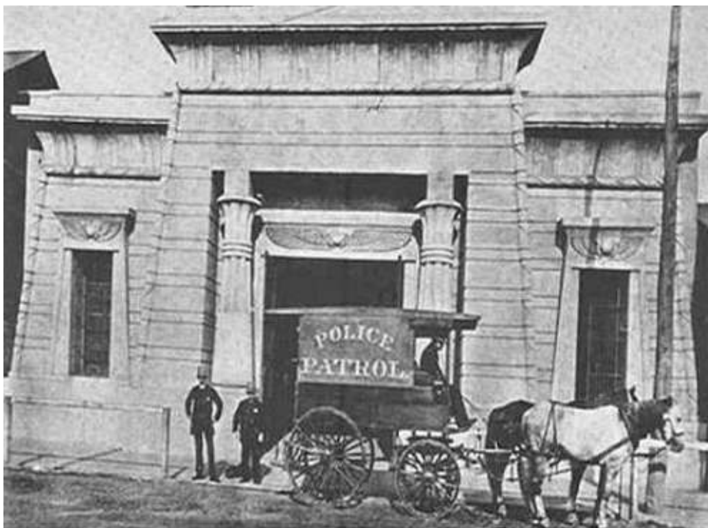
4th District Police Station on Rousseau Street in 1897, still there today
